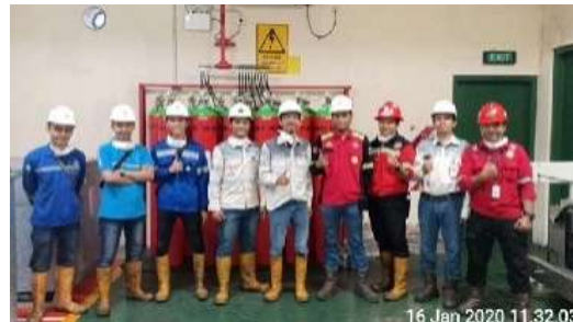
Fire Alarm & Clean Agen System CPBL PT Adaro Indonesia-Kelanis
